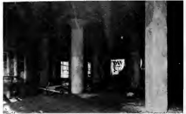
FIG. 6. APPEARANCE OF THE FLOOR AFTER FORMS WERE STRIPPED
